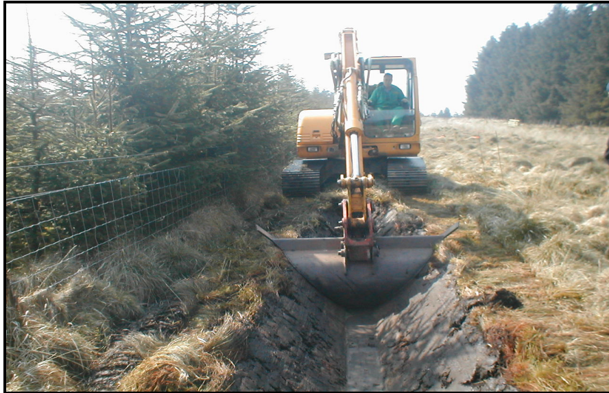
Figure 1. Cutting open drainage ditches by an excavator.
